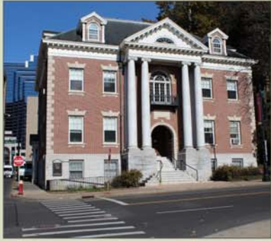
Church House at 60 Gold Street
